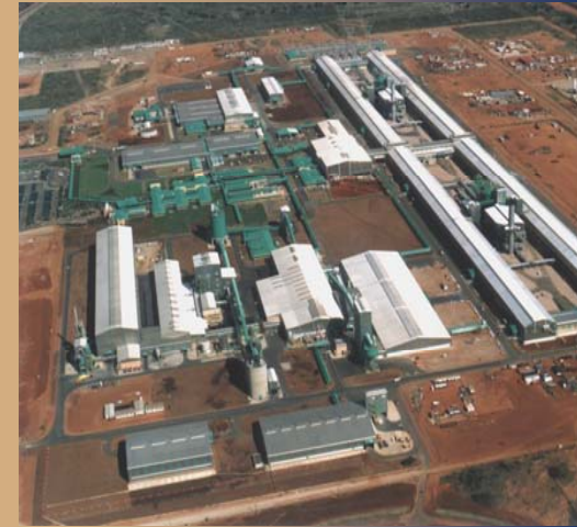
Mozambique Aluminium Smelter (MOZAL)
